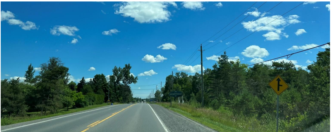
Figure 4: County Road 43, south of the subject site, looking east.
